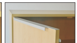
Aluminium handle protects top of door
